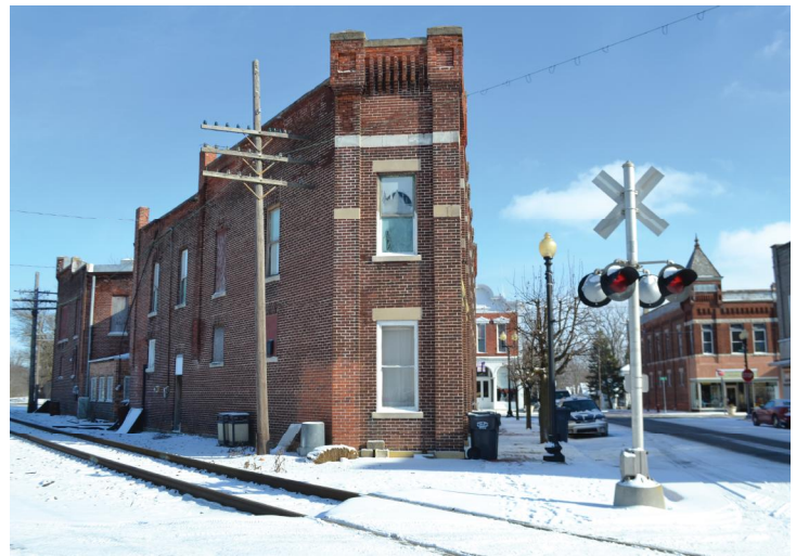
Historic Gray Hotel Building
