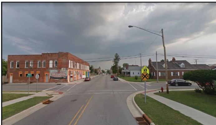
Meridian Street Corridor Looking South
