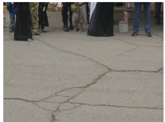
High Street Pavement
